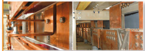
▶ ELEKTROLYSIS: BUSBARS
